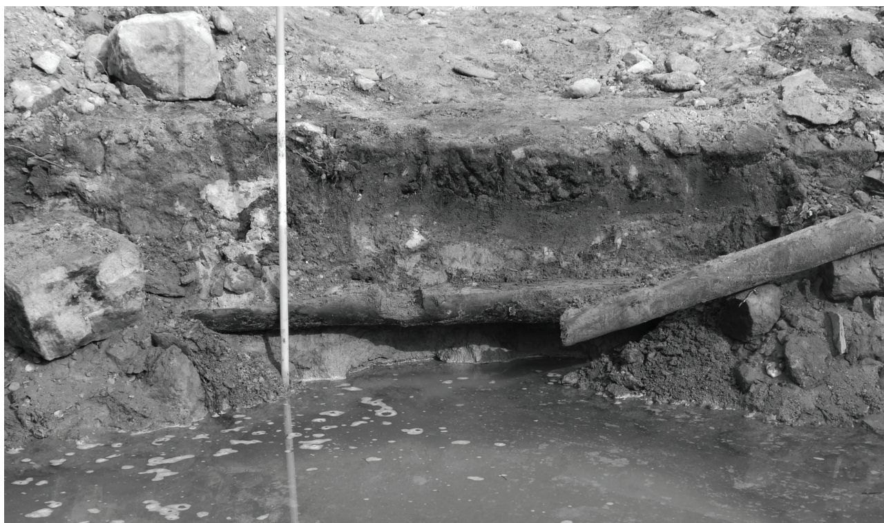
Fig. 17. Foundations of the bridge near the village of Žizníkov (source: VMG archive).
