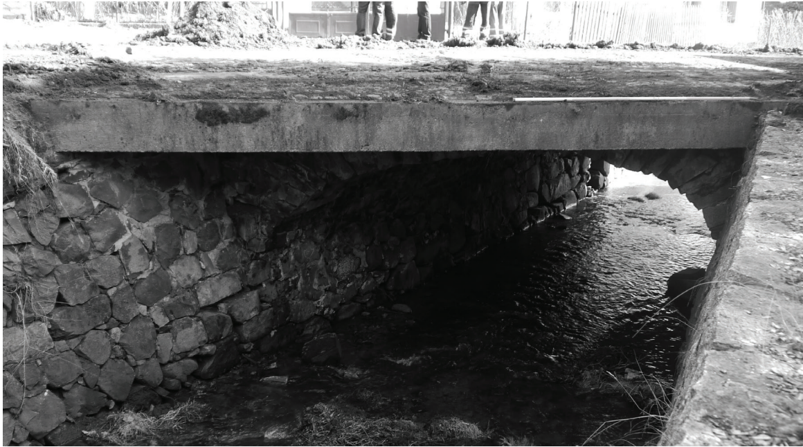
Fig. 10. Bridge in the city of Žandov (source: VMG archive).
