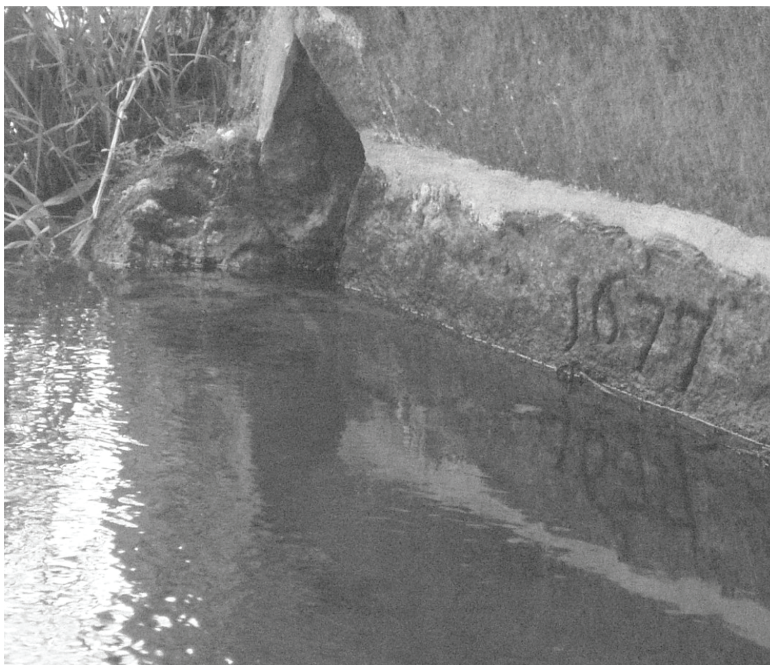
Fig. 14. Dating "1677" on the bridge in village of Velenice (source: VMG archive).
