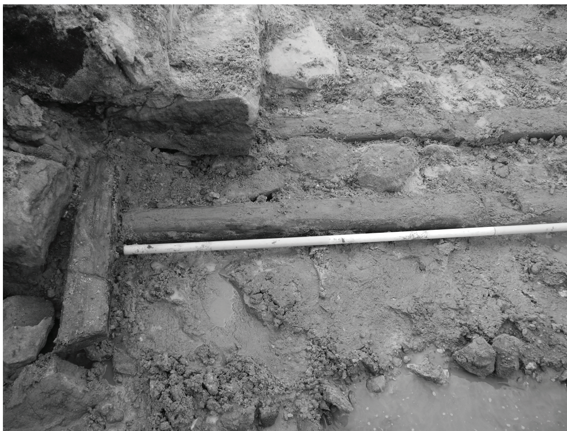
Fig. 19. Foundations of the bridge near the village of Žizníkov (source: VMG archive).
