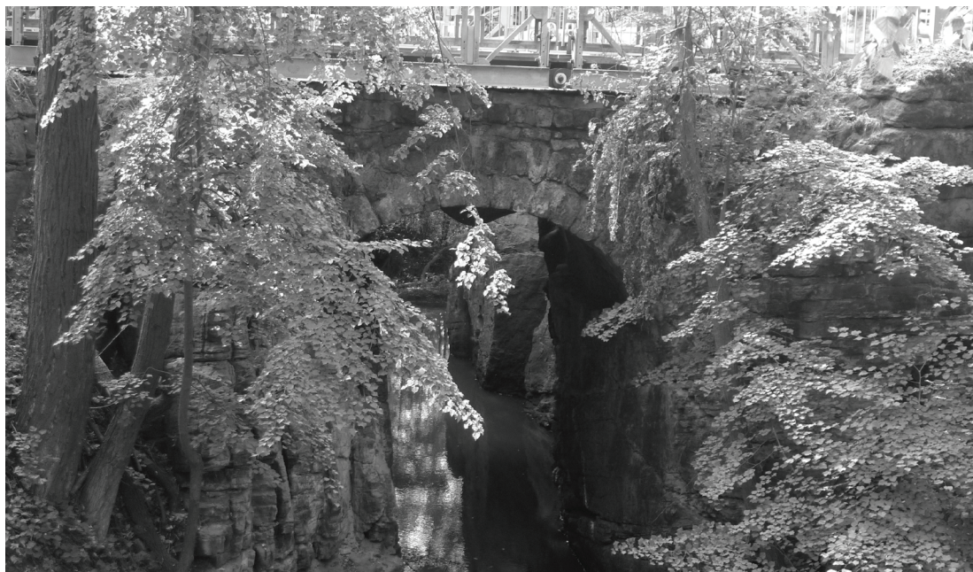
Fig. 13. Bridge over the Munich gap in the village of Zahrádky (source: VMG archive).
