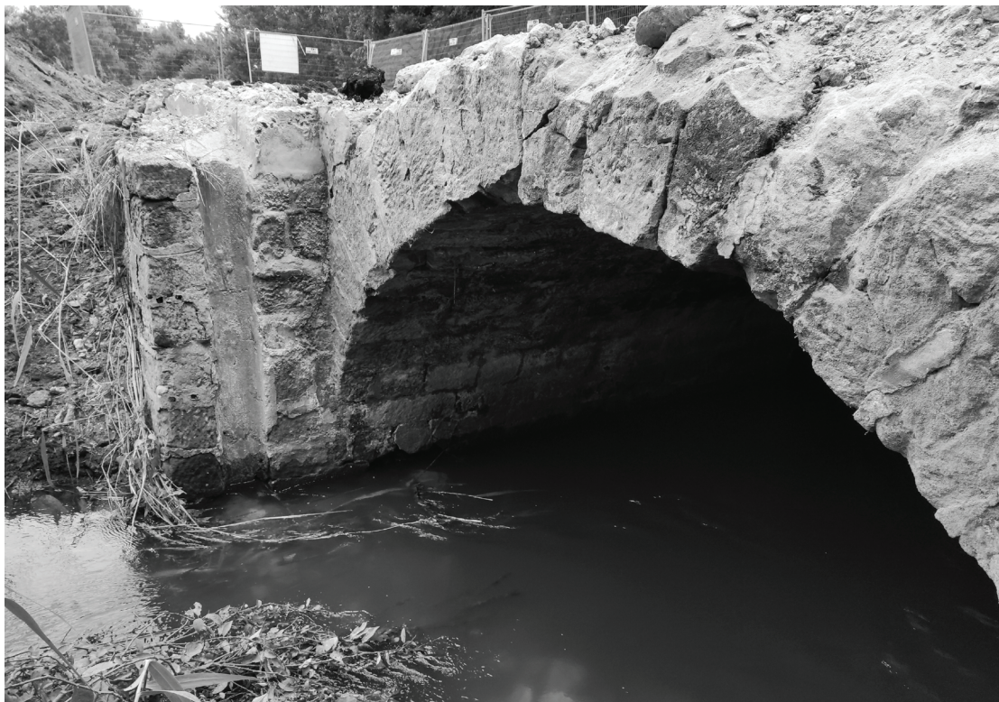
Fig. 6. Front view of the bridge vault on the upstream side with a groove used for waterflow regulation (source: VMG archive).
