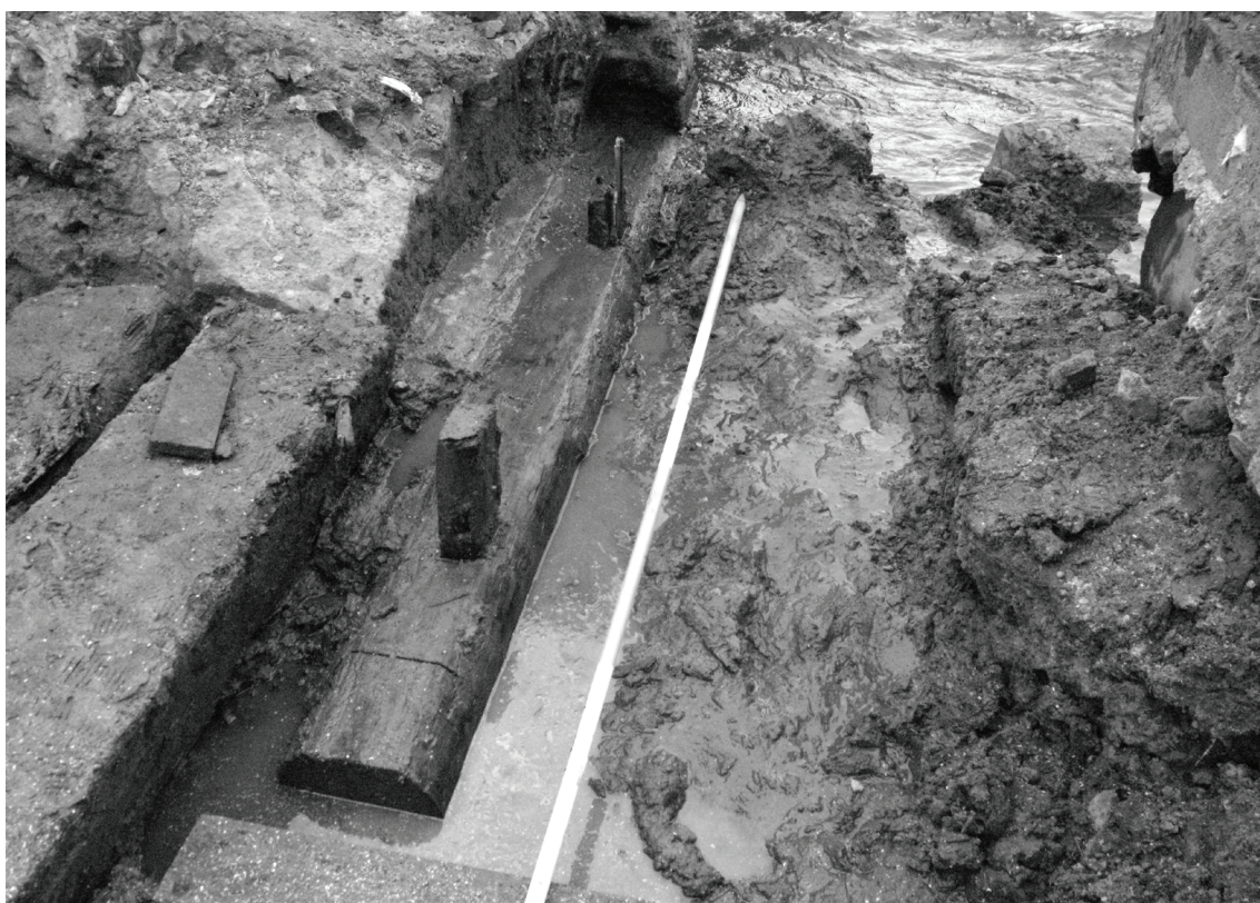
Fig. 21. The foundation of the 3 rd bridge pillar of the Zámecký (Castle) bridge (source: VMG archive).
