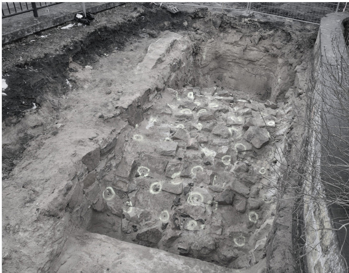
Fig. 11. Revealed construction of the oldest part of the bridge over Novozámecký gap in the village of Zahrádky (source: VMG archive).
