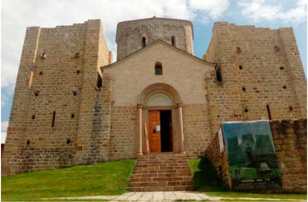
Fig. 4. Church of St. George, Monastery of Đurđevi Stupovi, 12 th century, view from the west (Photo by O. Špehar)
