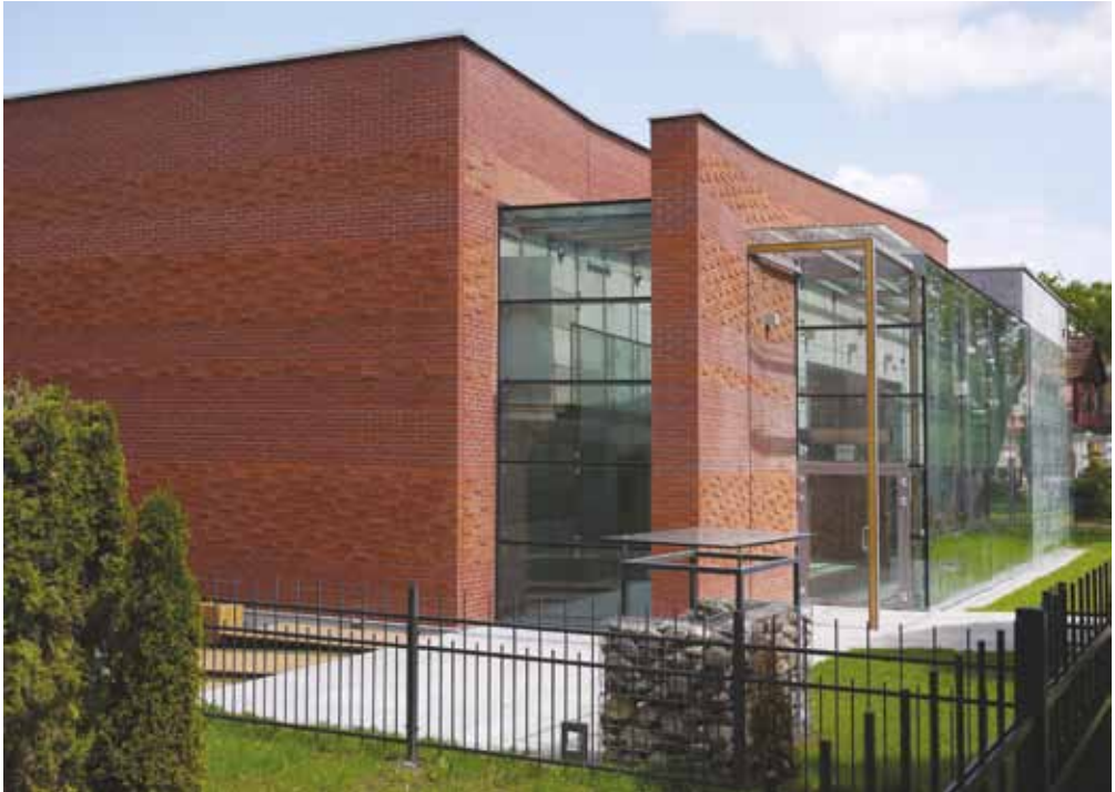
Fig. 4. The building which houses the Genius Loci Archaeological Reserve (Photo by K. Zisopulu-Bleja)
