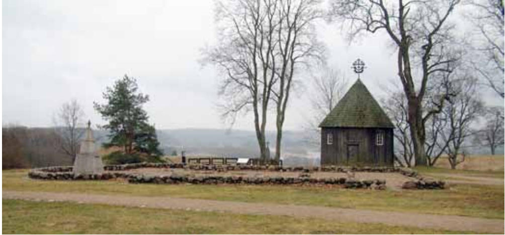
Fig. 12. Foundations of the church in Kernavė (1739): in situ visualisation (Photo by D. Vaičiūnienė; Collections of the Administration of the State Cultural Reserve of Kernavė)
