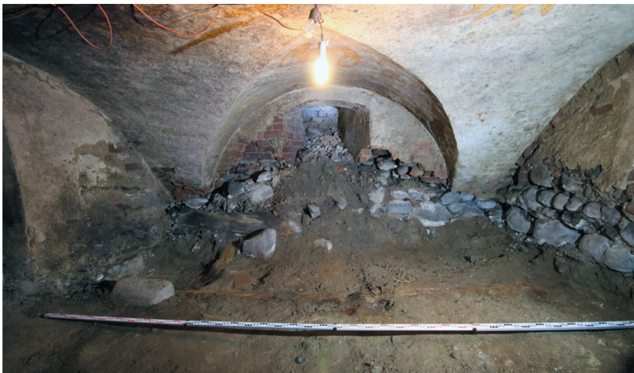
Fig. 3. The crypt's eastern wall: with a ventilation-light opening, the wall's destruction and original wooden joists visible in the crypt pugging. Photo by S. Nowak.
