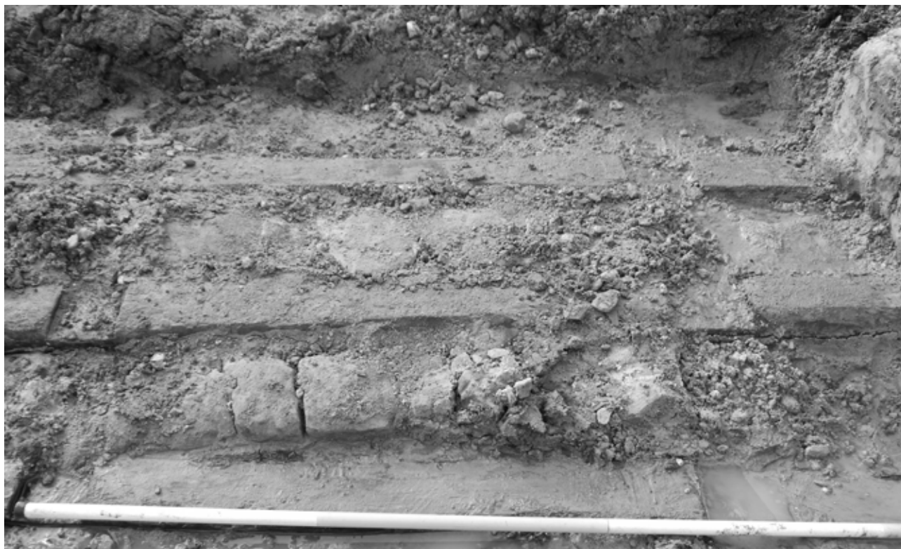
Fig. 18. Foundations of the bridge near the village of Žizníkov (source: VMG archive).
