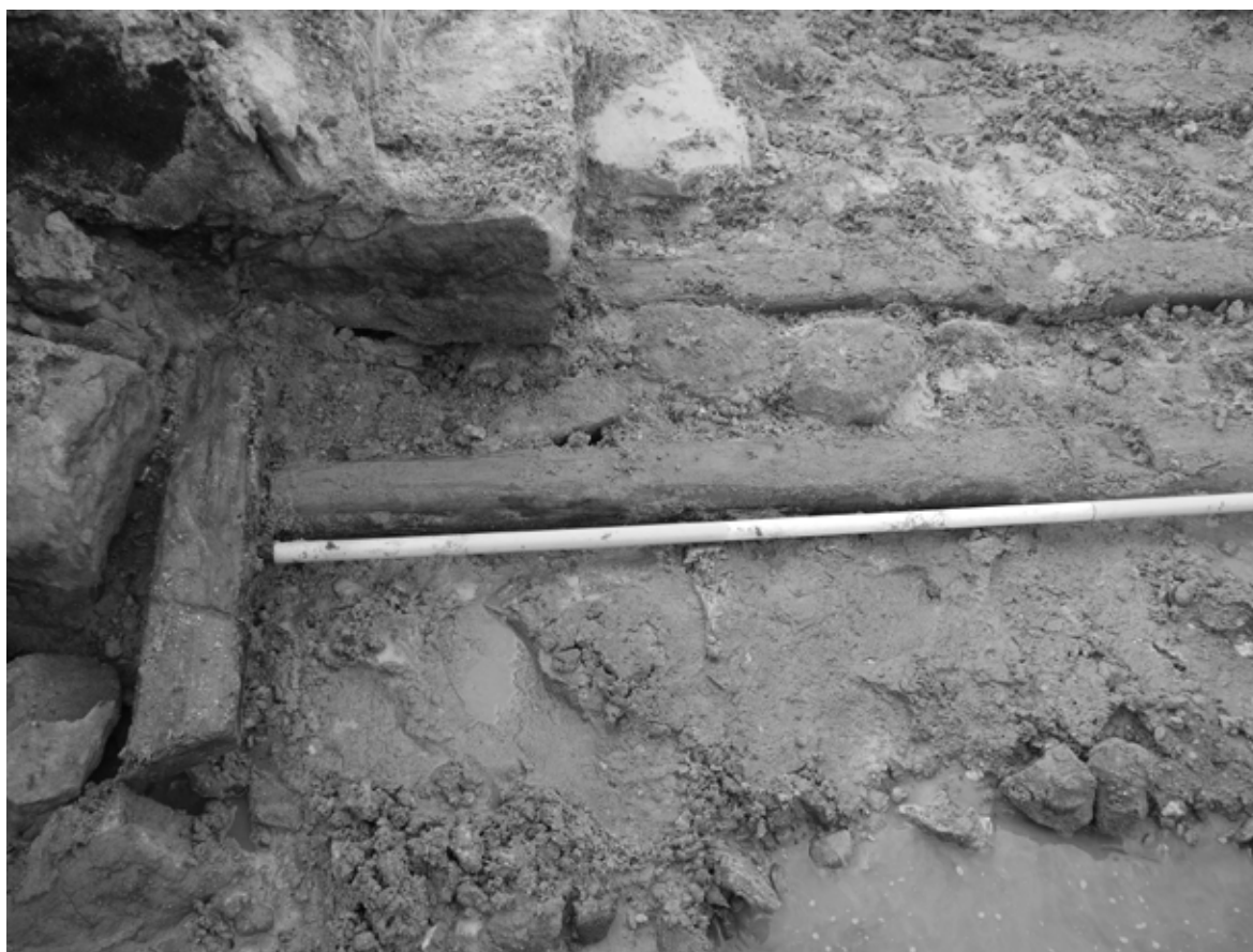
Fig. 19. Foundations of the bridge near the village of Žizníkov (source: VMG archive).
