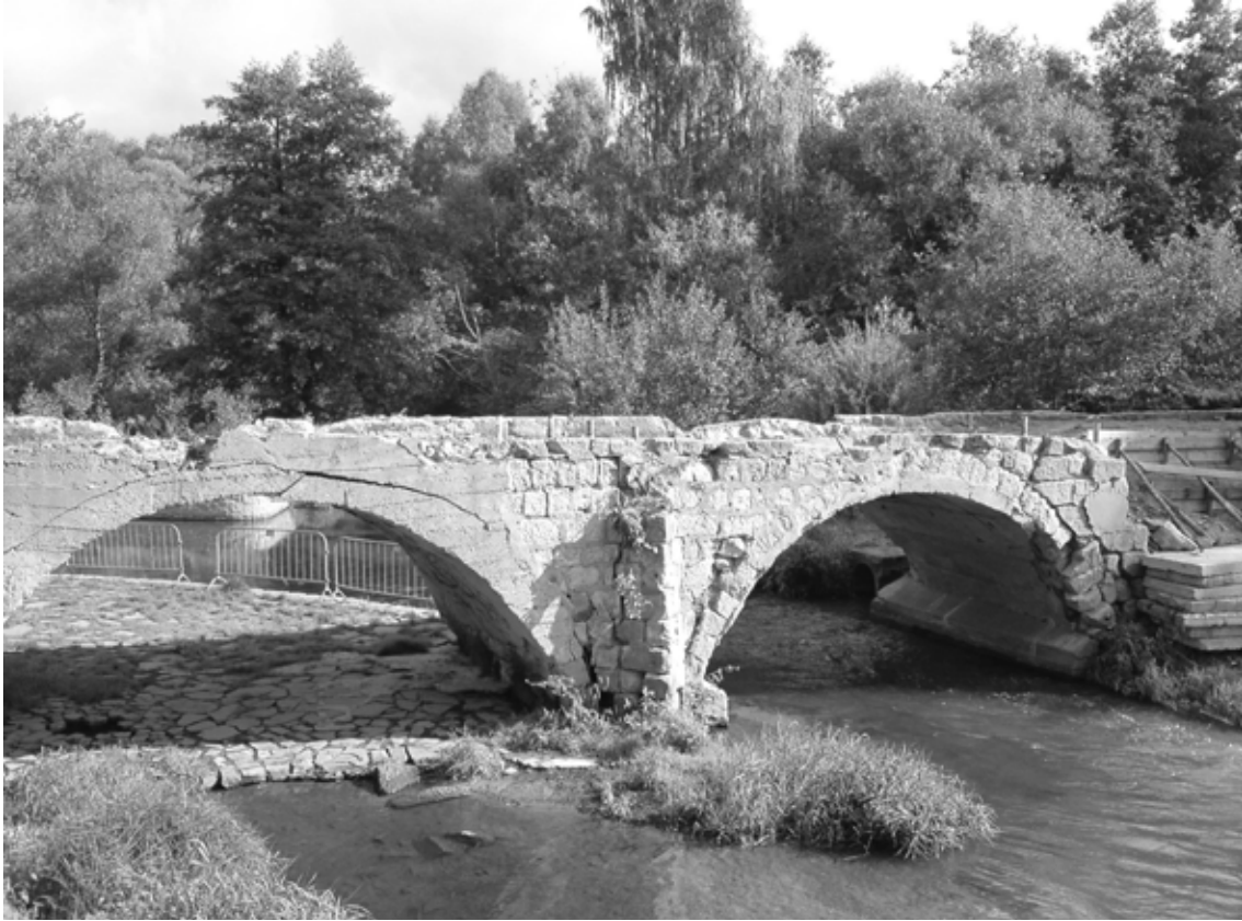
Fig. 20. View of the central part of the Zámecký (Castle) bridge in a prereconstruction state, city of Mimoň (source: VMG archive).
