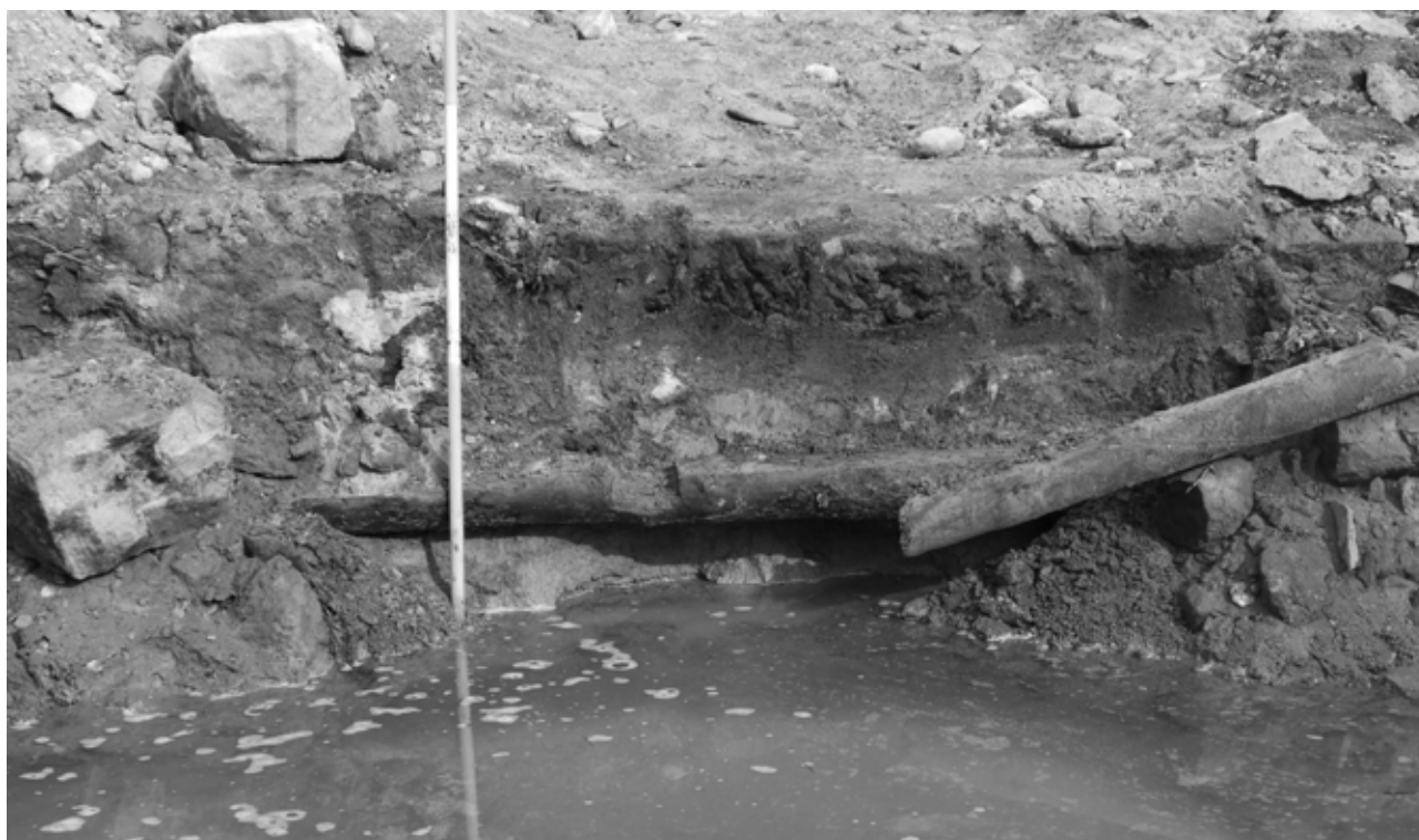
Fig. 17. Foundations of the bridge near the village of Žizníkov (source: VMG archive).
