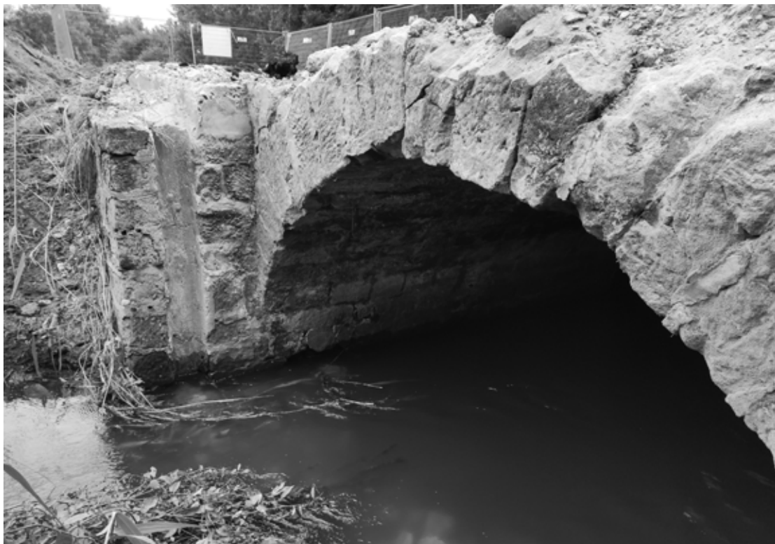
Fig. 6. Front view of the bridge vault on the upstream side with a groove used for waterflow regulation (source: VMG archive).
