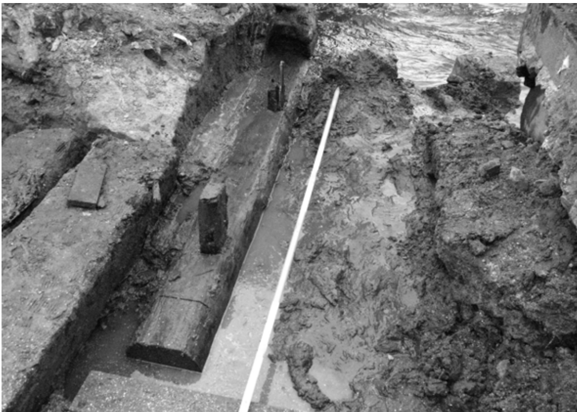
Fig. 21. The foundation of the 3 rd bridge pillar of the Zámecký (Castle) bridge (source: VMG archive).
