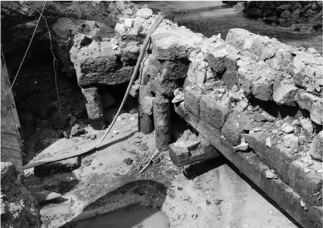
Fig. 7. View of the uncovered individual piles and grid beams under the abutment on the left bank of the stream. In the front right, a short transverse beam with mortises that were not used in the bridge construction (source: VMG archive).
