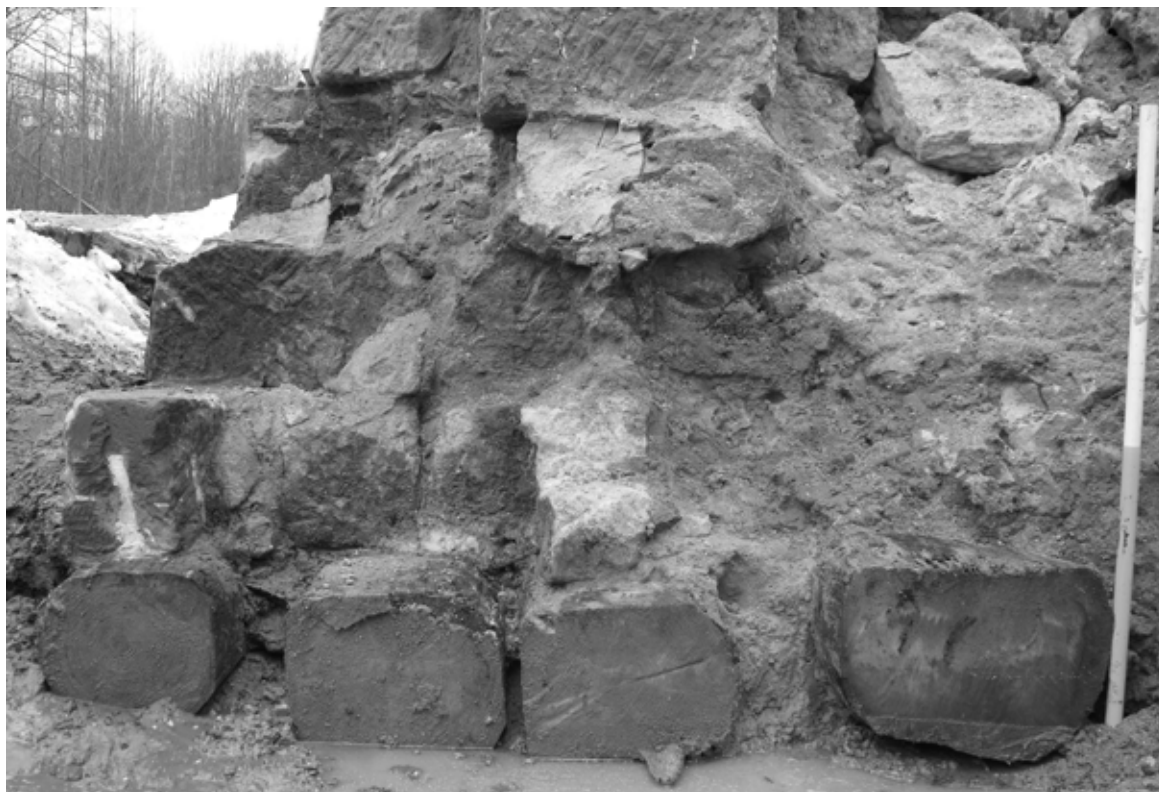
Fig. 22. The foundation of the 3 rd bridge pillar of the Zámecký (Castle) bridge (source: VMG archive).
