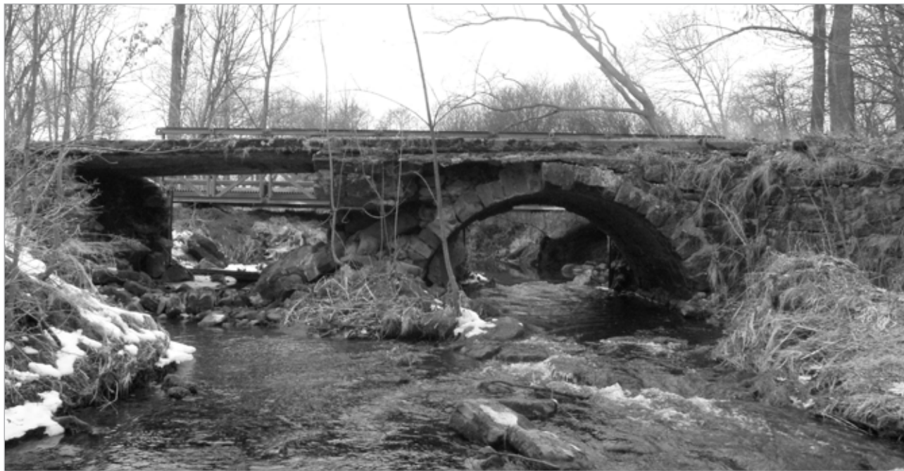
Fig. 15. Bridge in the village of Stvolínky (source: VMG archive).
