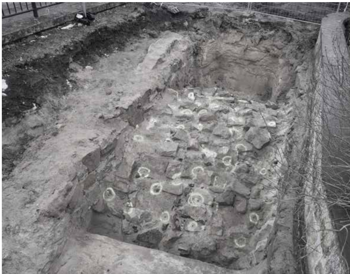
Fig. 11. Revealed construction of the oldest part of the bridge over Novozámecký gap in the village of Zahrádky (source: VMG archive).
