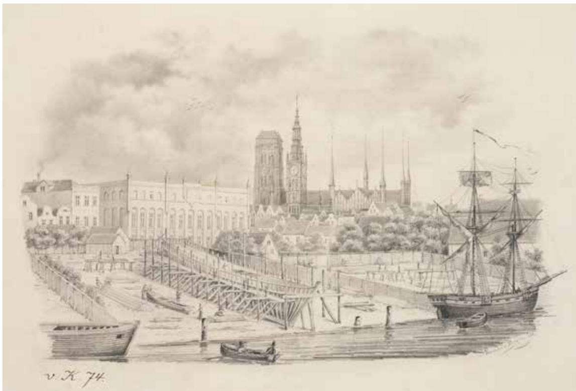
Fig. 7. Engraving from 1846 showing the Bordingfeld – a part of the Gdańsk Lastadia presenting the moment of construction of a wooden ship being prepared for launch with the bow towards the water (from the collections of the National Museum of Gdańsk).
