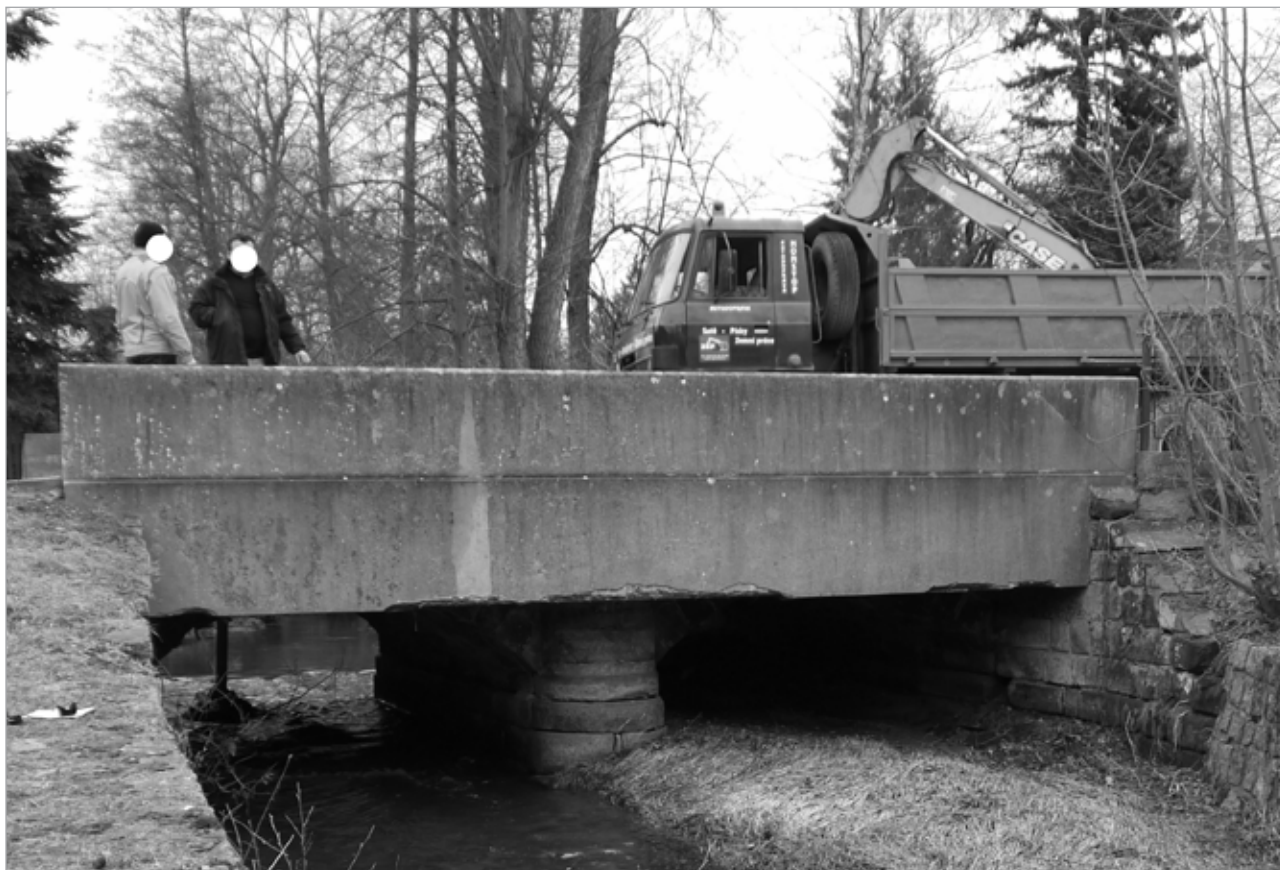
Fig. 16. Bridge in the village of Sloup v Čechách (source: VMG archive).
