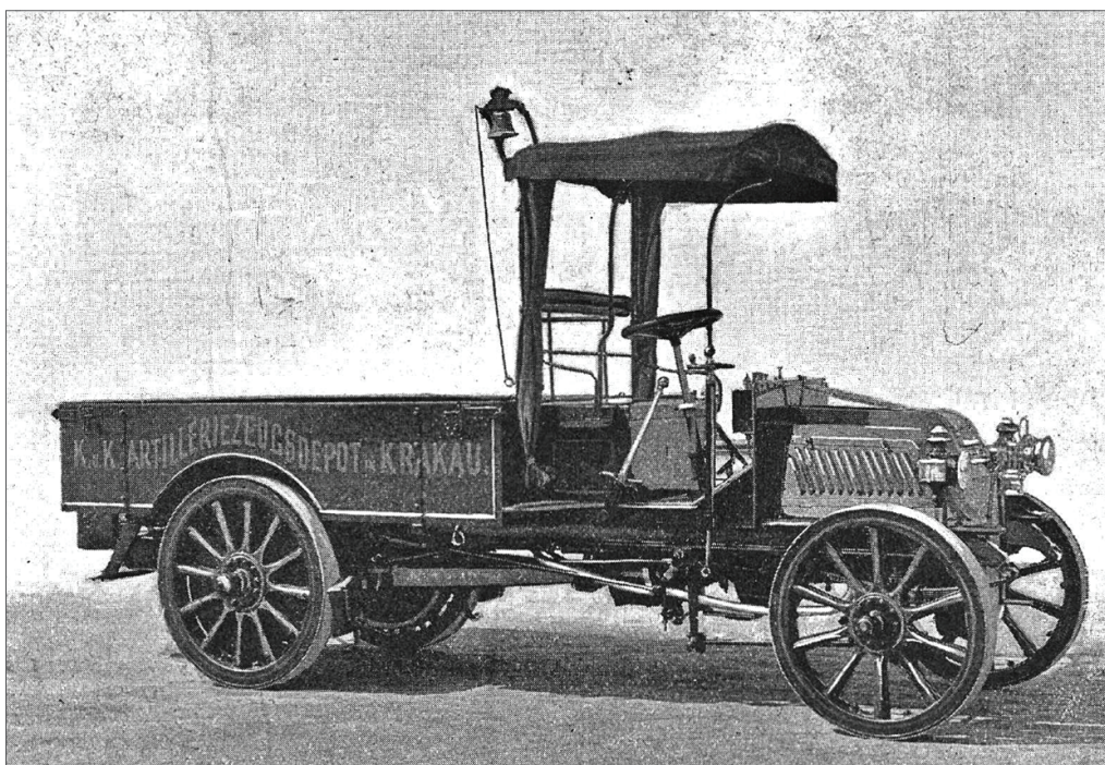
Phot. 7 One of the first two military Daimler 12/14 HP trucks, which appeared in Cracow in 1903. The car shown in the illustration belonged to K.u.K. Artilleriezeugsdepot in Krakau. ("Allgemeine Automobil-Zeitung" no 18 of 1.V.1904, p. 17)
