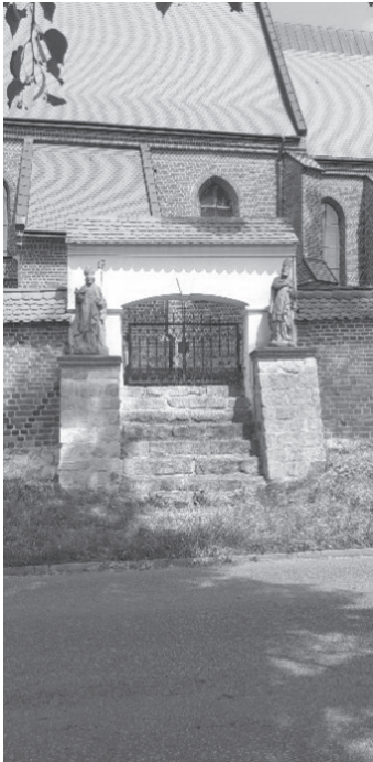
Photograph 2. Contemporary view of the former entrance.
